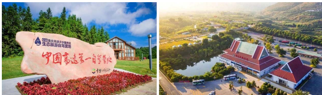
图 1 冷水服务区、潞江坝服务区 Fig.1 Lengshui Service Area and Lujiangba Service Area
