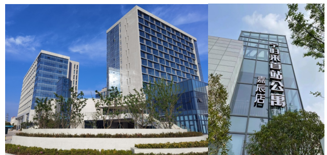
图 2 南京“宁归来首站公寓” Fig.2 "Ningguilai First Station Apartment" in Nanjing
