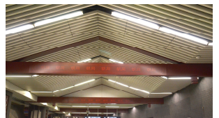
图2 室内吊顶1 Fig.2 Interior ceiling 1
